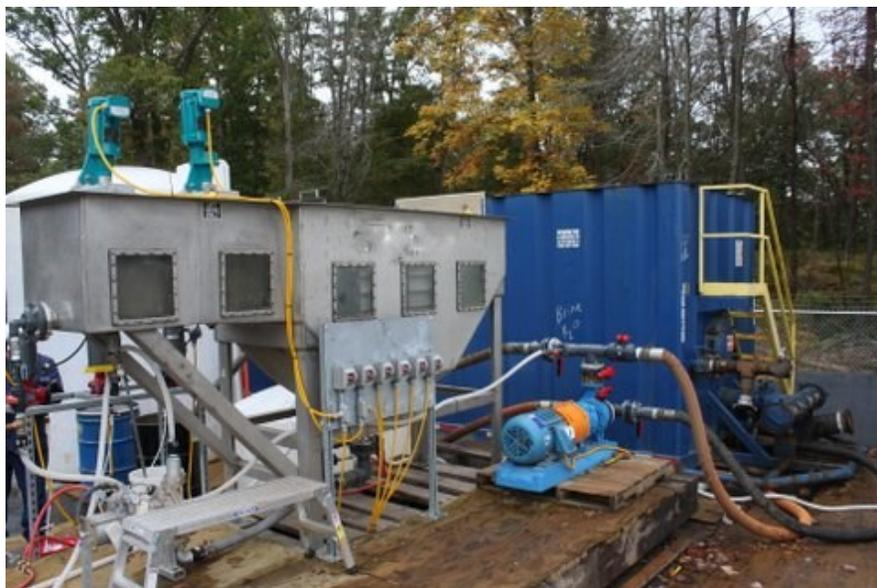
Frack tanks were used for equalization to the feed system.
