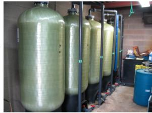
The challenge was to do a replacement of the steel retention tanks and re-bed both softeners without shutting down the travel center's operations. This facility provided showers for drivers as well as supplied two different restaurants. The goal was to provide potable water to maintain these functions plus meet fire suppression requirements.
