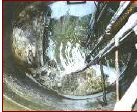
After 6 weeks of treatment with FOG 2000: 90% of the lift station water has no grease cap. The tan color areas on top of the grease show the grease is thinner and has not been in the station for long periods of time.
